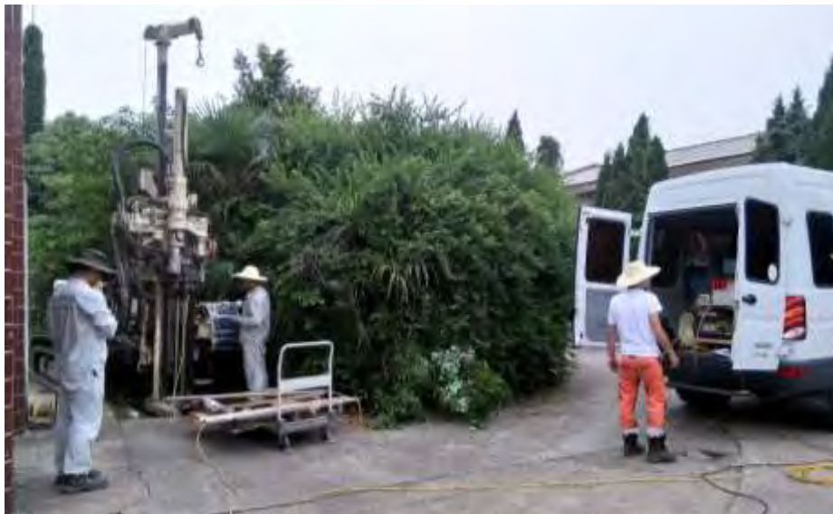
Figure 2: Ejlskov drilling operations and set up performing MIP surveying
